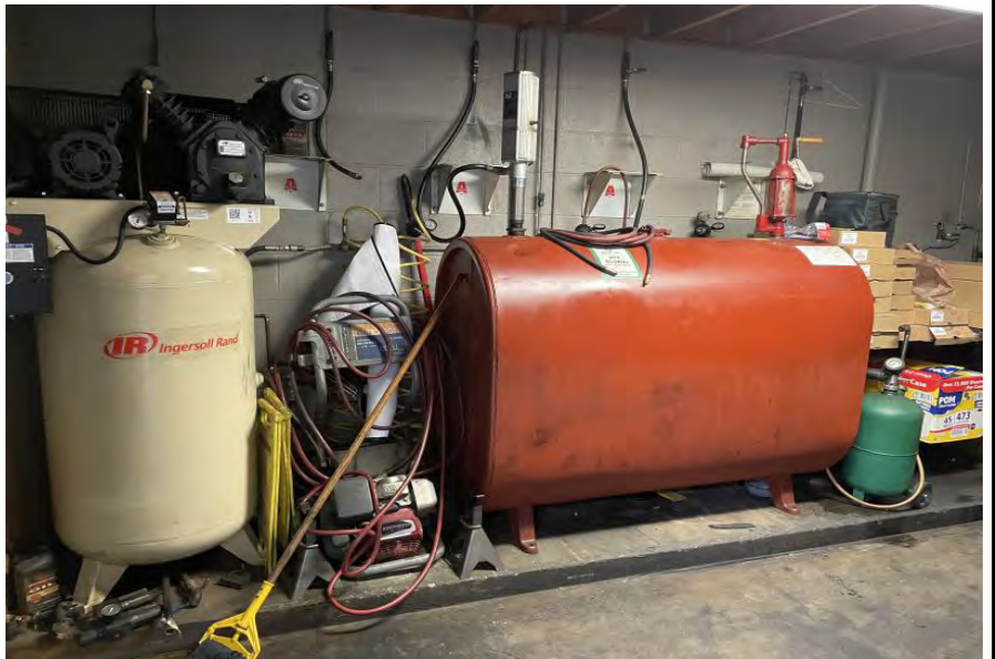
Photo 14 Lube Shop Aboveground Storage Tank
