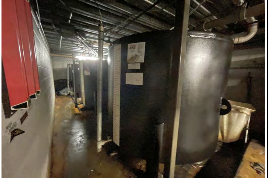
Photo 13 Lube Shop Aboveground Storage Tank
